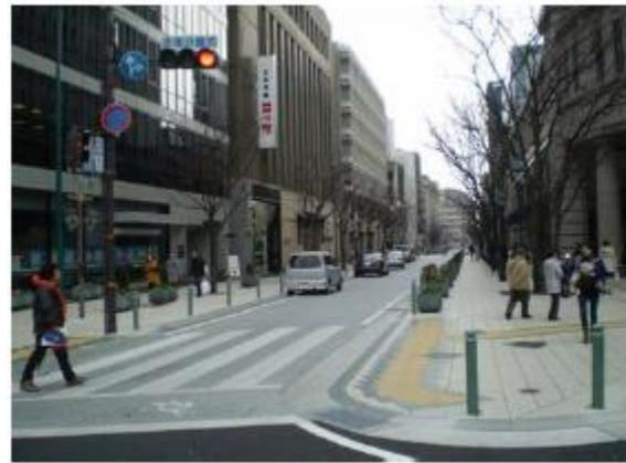
写真-3 遮熱性舗装(車道)と透水性舗装(歩道)
